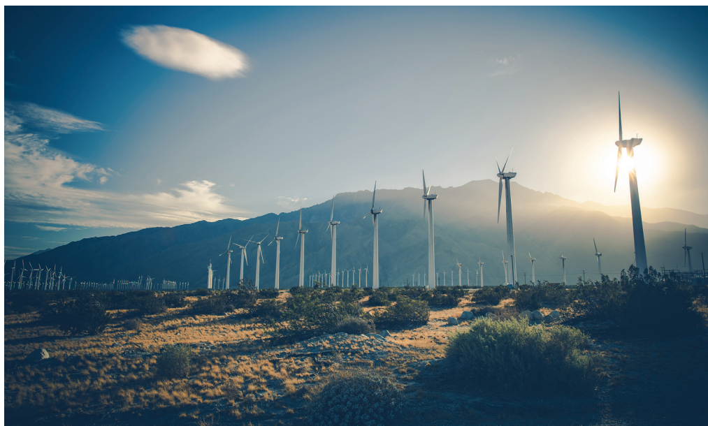
California Renewable Energy. Wind Energy Power Plant. Coachella Valley, United States of America. © Welcomia | Dreamstime.com
